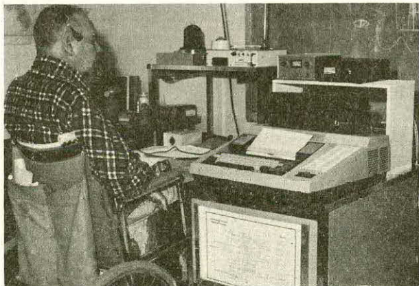
Figure 1. Voice-Operated Typewriter and Environmental Control System
